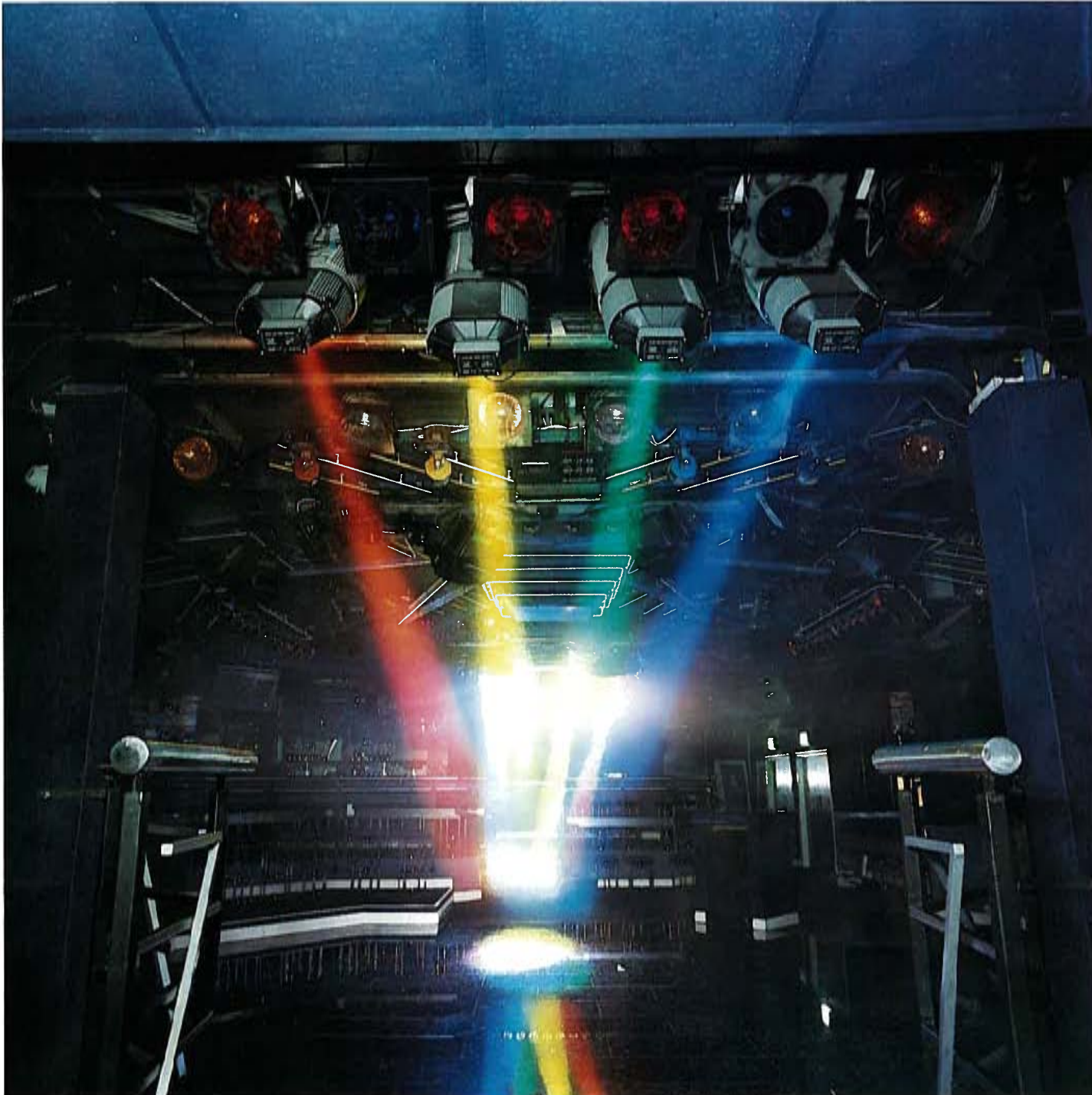
A close-up of the first UK installation of Clay Paky Golden Scans.
