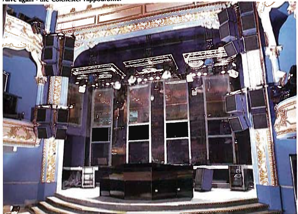
Balcony and dance floor sound: two vertical clusters, each comprising six Turbosound TSE-111's and four TSE-115's, hang on either side of the proscenium arch.
