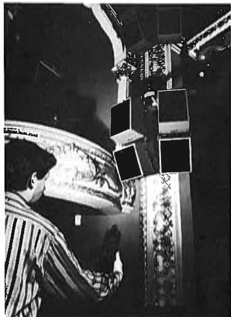
Electromusic's Scanalyser being used to check the Hippodrome's sound system.
